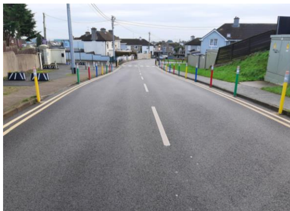
Figure 17-4 Completed SRTS scheme at SS Michael and Peter Junior N.S. on St Mary's Road Source: WCC.
