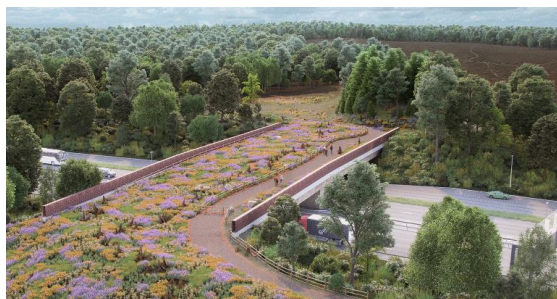
Figure 10-4 CGI of the Cockcrow Bridge (under construction as of Q1 2025), which will reconnect two heathlands at either side of the M25 motorway. Source: National Highway.
