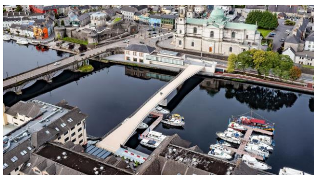
Figure 10-3 Example of an active travel bridge over the River Shannon in Athlone. Source: Irish Times.
